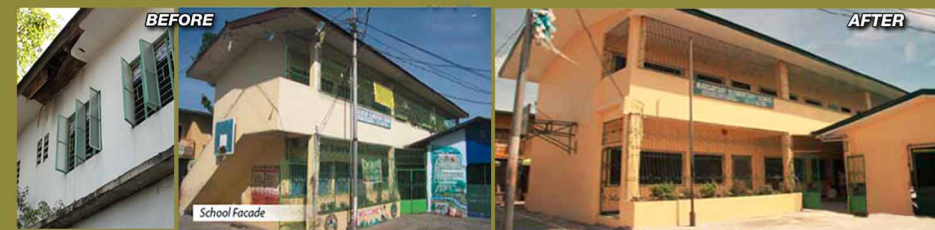
Renovation of Magsaysay Elem School Dau Mabalacat Pampanga.
